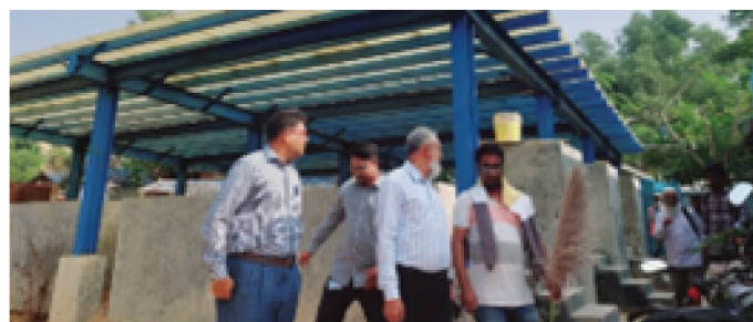
Fecal sludge treatment plant at Rohingya Camp 12
