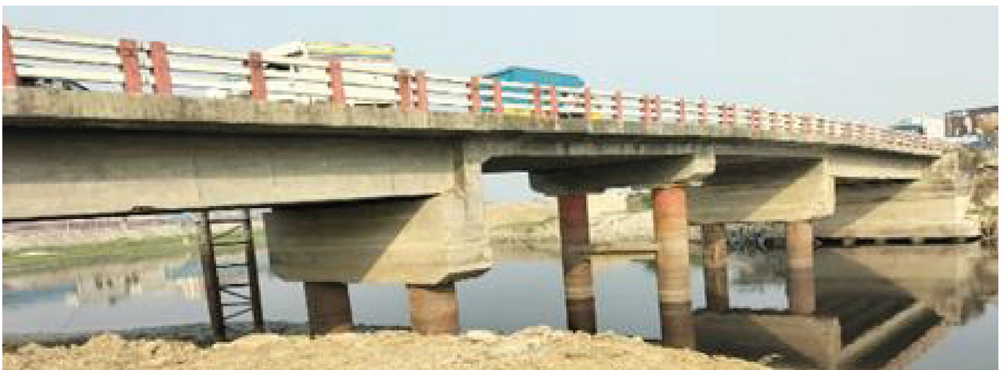
Bridge Over Inland Waterways
