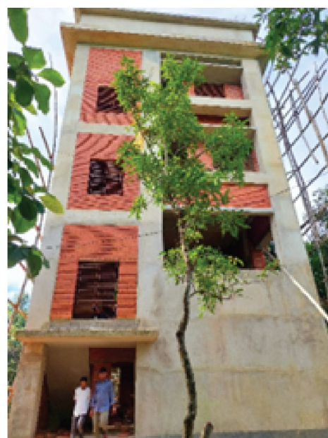
Water Treatment Plant for Host Communities
